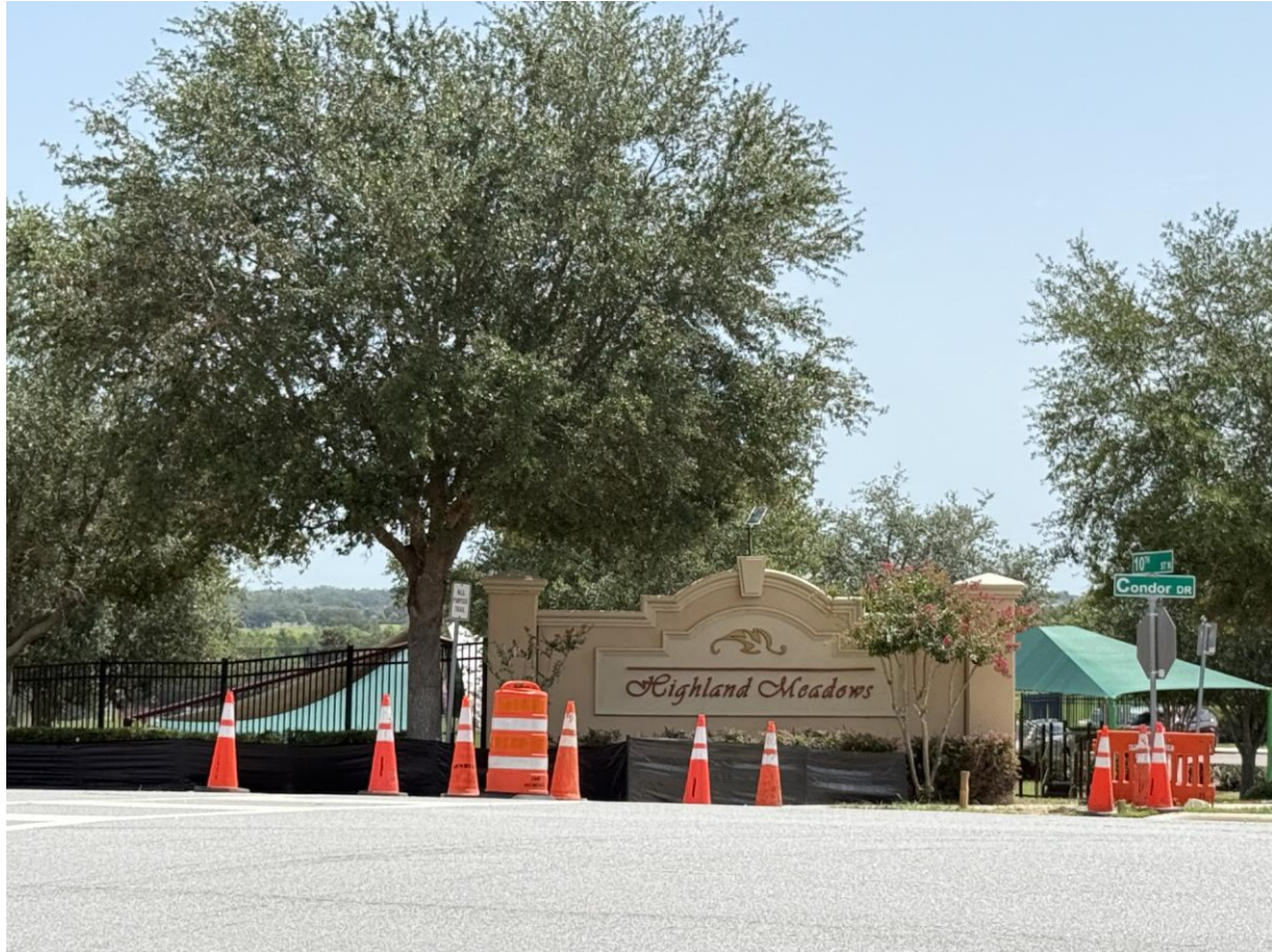
Construction going on outside of pool area
